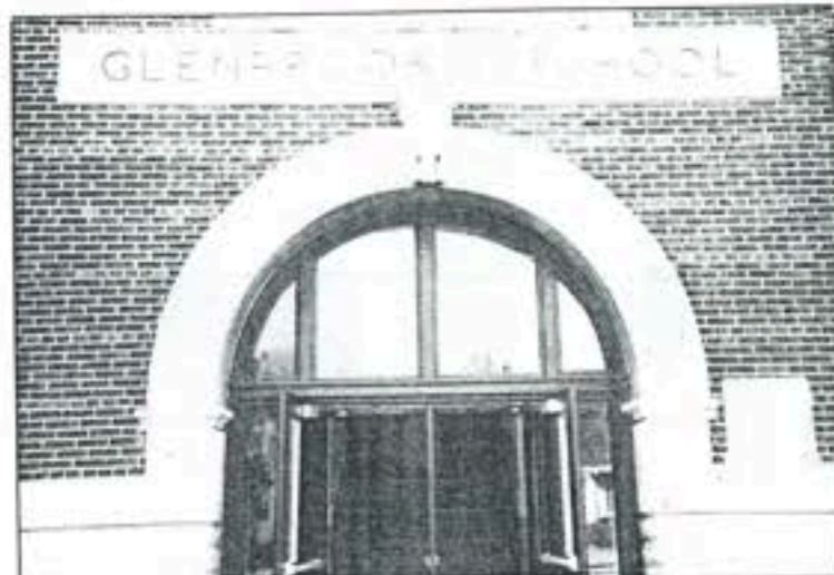
The archway will be preserved while the rest of the old High School will be torn down in June.
