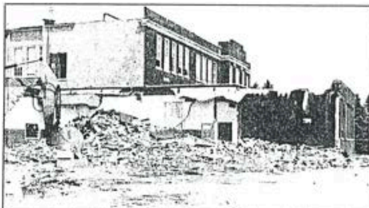
Wreckage from the old Glenbrook School lies where a new and improved facility now stands.
